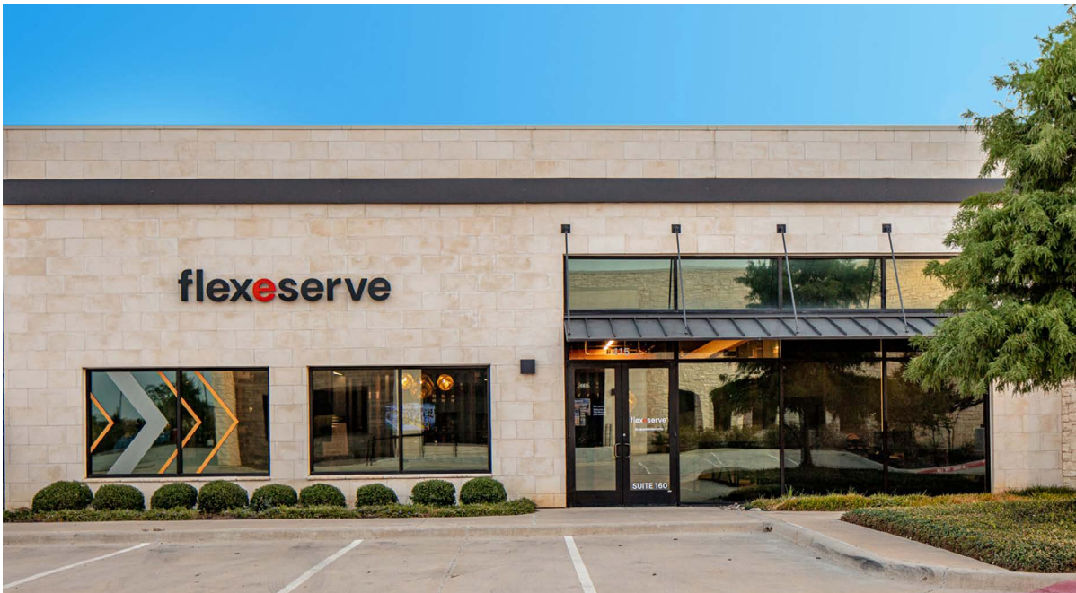
Flexeserve Inc.'s new HQ and Culinary Support Center in Southlake, Dallas TX
